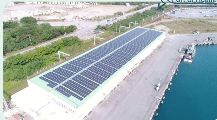
Warehouse No. 6, Port of Hualien
