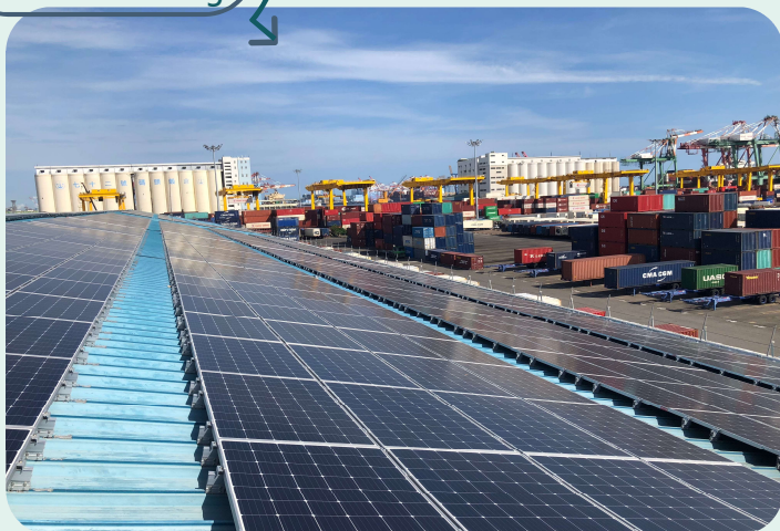
Third Container Terminal, Port of Kaohsiung
