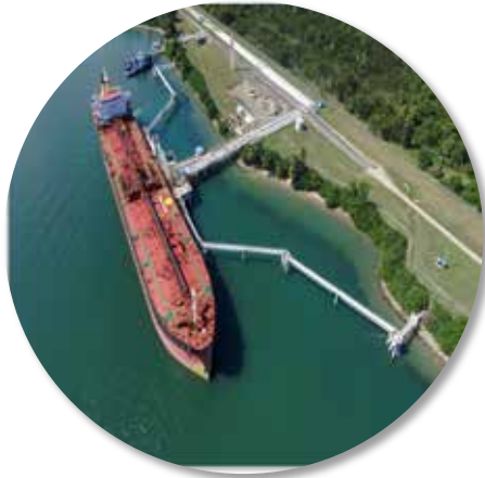
UAV / Drone Inspection
