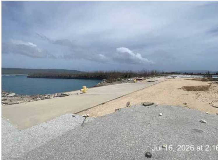
West Quay – RoRo Ramp
