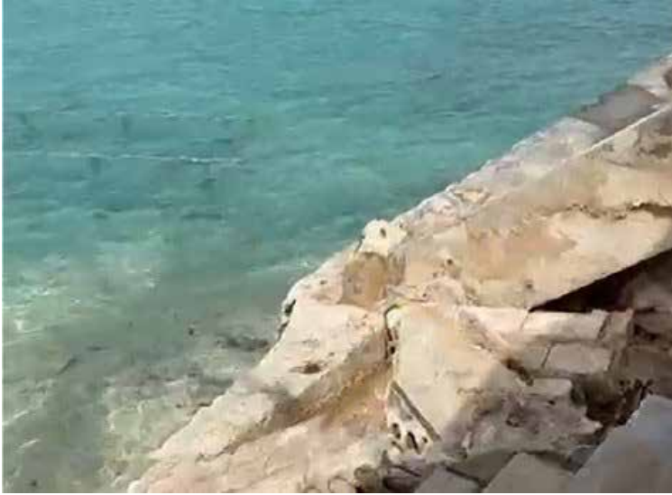
Storm-Damaged Steps
