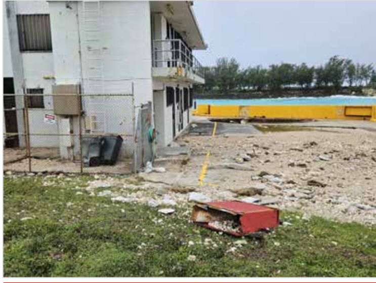
CPA Office at Berth 2
