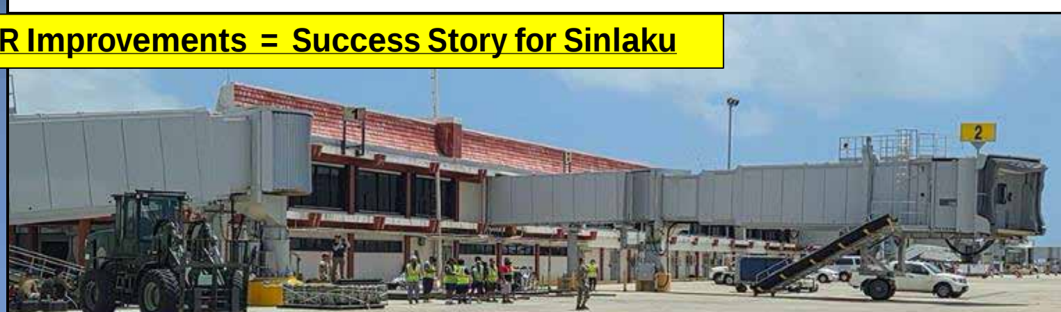
Jet Bridges were recently rebuilt to withstand typhoon level winds. Survived Sinlaku and were a receiving area for air response commodities.
